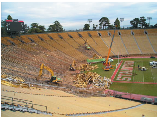
Ferma's task was to leave a smooth, clean earthen bowl for the dirt contractor to work with. >
